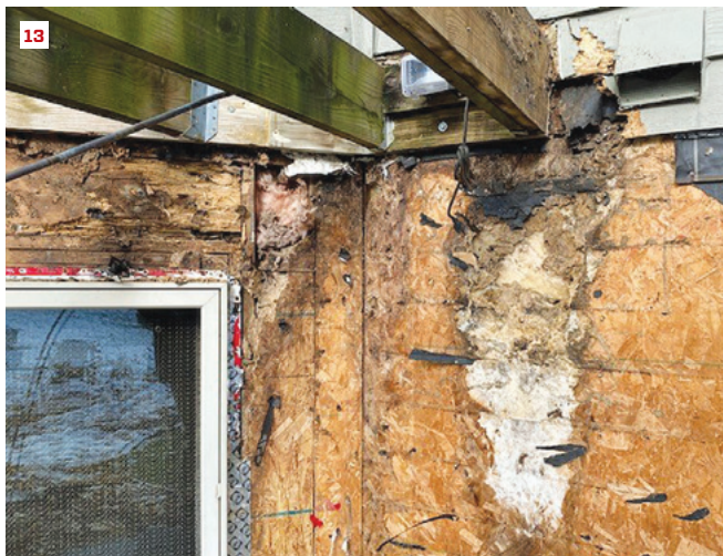
The flashing used for this deck ledger (13) was a site-bent aluminum L-flashing installed with steel nails. The dissimilar metal caused rapid corrosion of the flashing, allowing water to get behind the ledger and saturate the OSB sheathing, which began to rot. Mitered clapboards (14), if done well, are more durable than woven corners that leave vulnerable end grain exposed.
