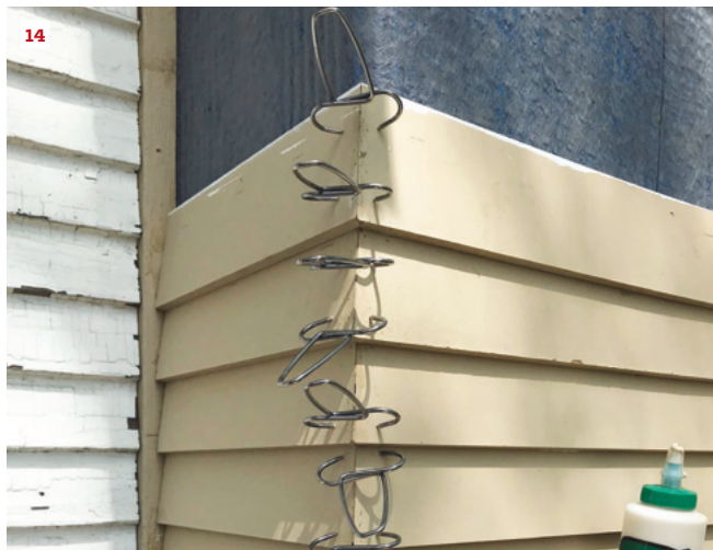
The flashing used for this deck ledger (13) was a site-bent aluminum L-flashing installed with steel nails. The dissimilar metal caused rapid corrosion of the flashing, allowing water to get behind the ledger and saturate the OSB sheathing, which began to rot. Mitered clapboards (14), if done well, are more durable than woven corners that leave vulnerable end grain exposed.
