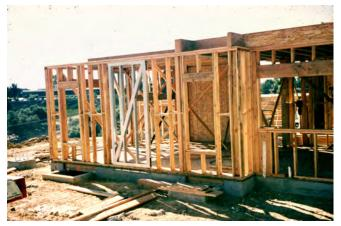
**Photograph 6: Shear Resistance**—Pre-manufactured metal inset shear panels are quite common in high seismic risk zones.
