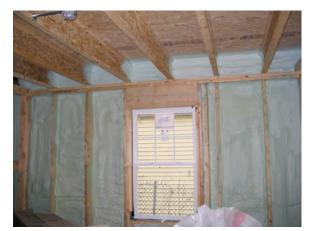
Photograph 5: High-Density Spray Foam Cavity Insulation—High tech and low perm. Great air sealing, great thermal performance, great structural strength. Does not allow for any appreciable inward drying of the exterior sheathing.
