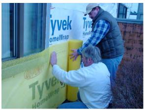
**Photograph 3: "High-tech air?"**—Polypropylene mesh providing an air gap between OSB covered with housewrap and cladding.
