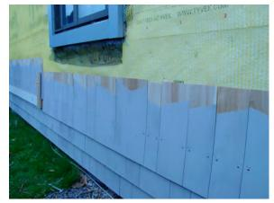
**Photograph 4: Cedar Shingles**—Back ventilation and drainage of wood shingle cladding installed over OSB covered housewrap – it does not get better than this from a durability perspective.
