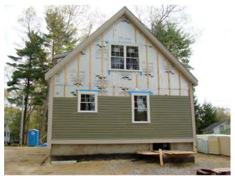
**Photograph 7: Furring**—When foam sheathings exceed 2 inches in thickness 1x4 furring becomes necessary. This wall has 4 inches of foil-faced polyisocyanurate insulating sheathing installed over a 2x6 wood frame wall. The wood furring acts as the nail base for the fiber-cement cladding.
