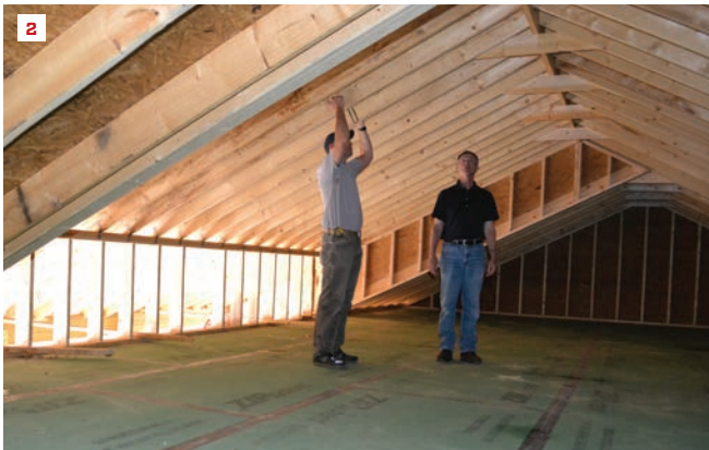
The Zip System sheathing on the attic floor creates a tight air seal (1). The stick-framed-attic volume is reserved for blown cellulose insulation, with no storage or equipment; here, the architect and builder discuss the ventilation strategy while they still have access to the space (2). Beneath the attic floor, the 2x10 joist cavities provide a convenient service chase that easily holds recessed lighting fixtures inboard of the air barrier (3). Continuous exterior insulation boosts the wall R-value (4).
